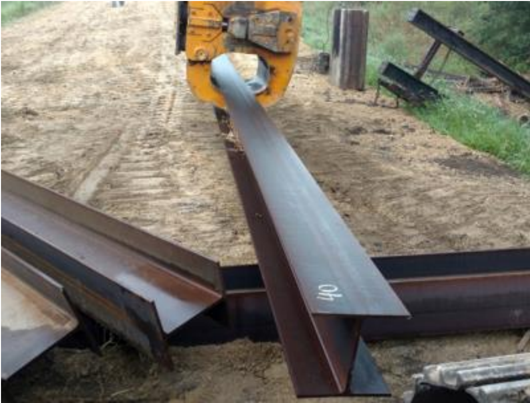
Loading a pile
